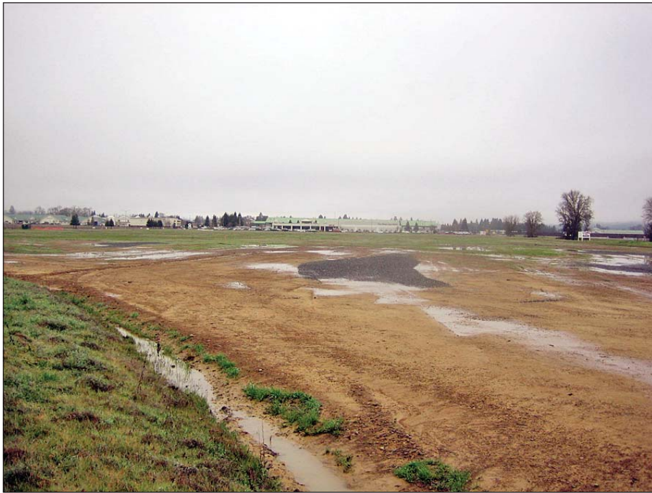
PHOTOGRAPH 3. Looking north from the south end of the project site.
