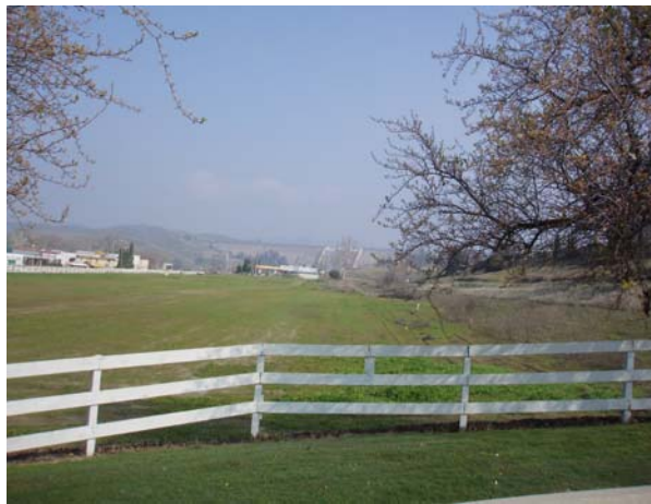
Looking north toward Friant Dam.
